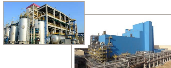
Mechanical completion of new production plants
