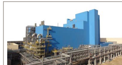
Superabsorbents plant (Al Jubail, Saudi-Arabia)
