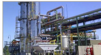
Alcoxides plant (Puerto General San Martin, Argentina)
